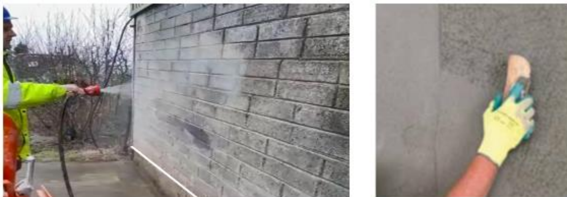
Figure 8 - Checking background suction and application of Super Bond
